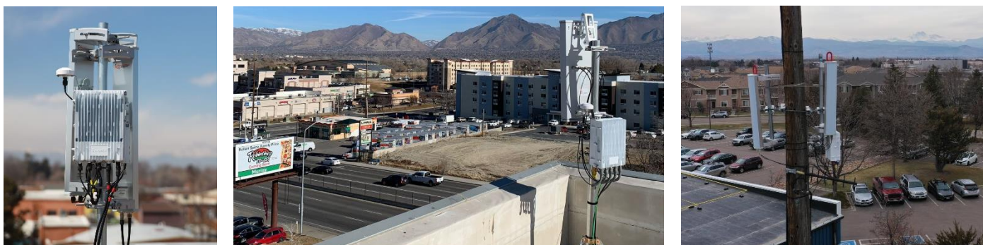
Fig. 3 – Small Cell deployments on rooftops of school district buildings
